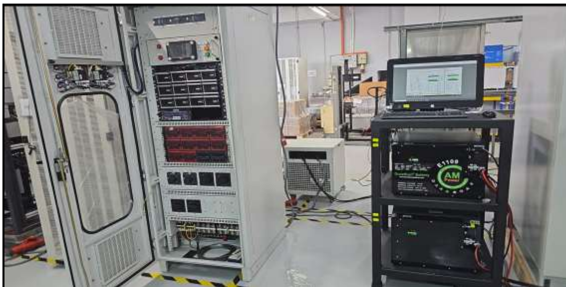
HPMI modular ups with Sodium Nickel chloride battery
